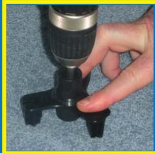
Using the driver bit provided, drive the screw down as far as the fixture will allow.
